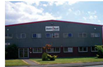
Production facility in Birmingham
